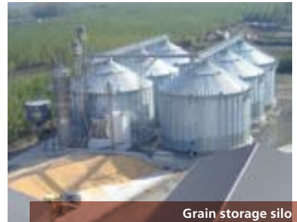
Grain storage silo
